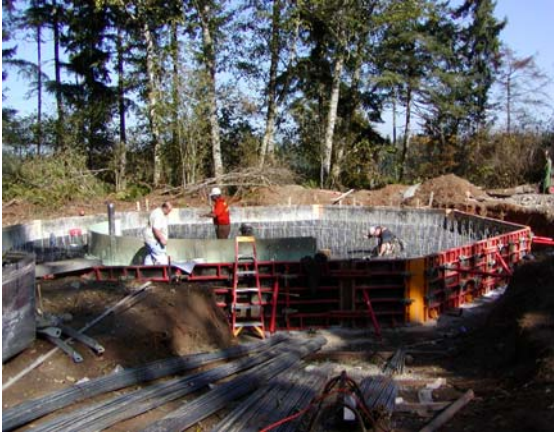
Water System Upgrade and Expansion, Nisqually Indian Reservation, Washington
