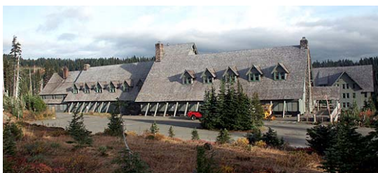
Drainage Improvements, Paradise Inn, Mt. Rainier National Park, Washington; Fletcher Farr Ayotte for the National Park Service
