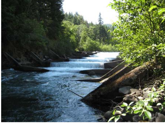
Moving Falls Fish Ladder and Trap Project, Confederated Tribes of the Warm Springs Reservation, Oregon
