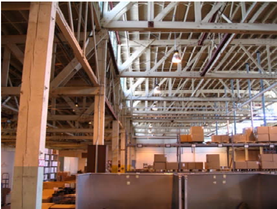
Ft. Lewis Timber Roof Truss Inspection, Ft. Lewis, Lacey, Washington
