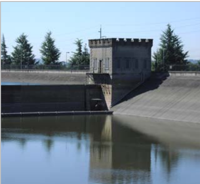
Historic Structures Reports, Mt. Tabor and Washington Park Reservoirs, Portland, Oregon
