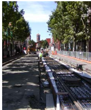
Portland Mall Revitalization Light Rail Project, Portland, Oregon; URS for Tri-Met
